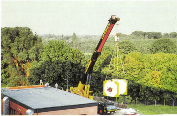
Fig. 1. The photograph shows the superconducting 4-T magnet — weight 50 tonnes — being lowered through the roof of one of the MR-research buildings at the Philips Hamburg laboratories.
